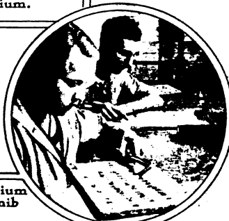
The 14K gold nib is tipped by hand with the hardest native iridium.
